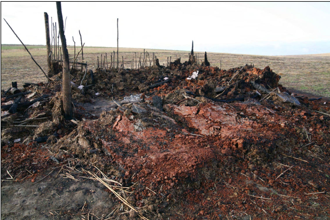
Photo 12. "Casa Bucovina" ( Bucovina House ) the next day after the fire. Zvoriștea 2008.
