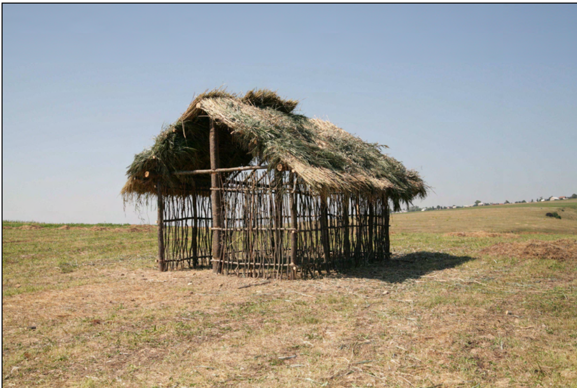
Photo 6. "Casa nordului" ( House of the North ) under construction. Zvoriștea 2008.
